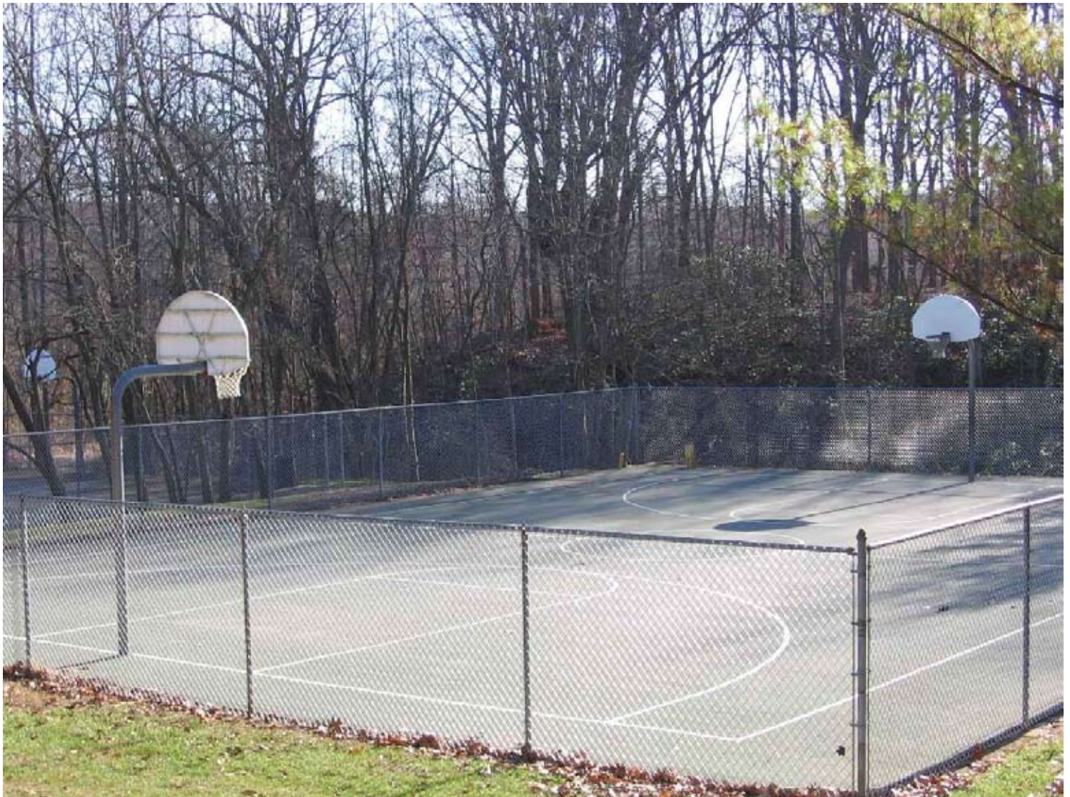
A view of the Bay Hills basketball courts with new fencing.
